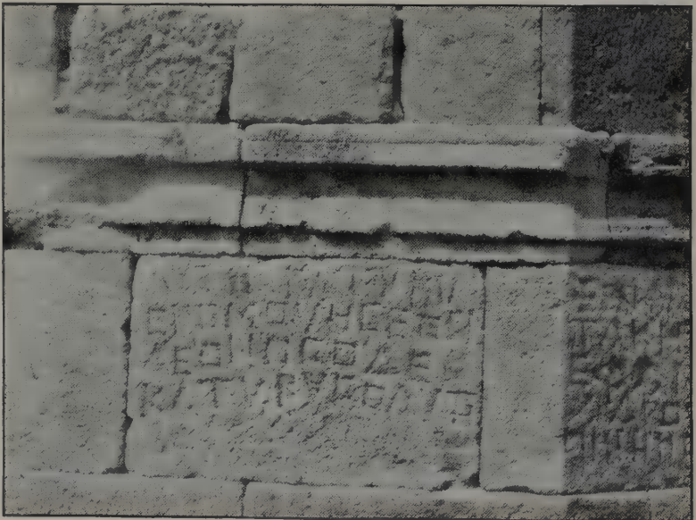
FIG. 15.—No. 3, moulding on outside of apse.
